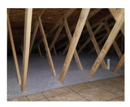
• Add 11" of blown cellulose insulation (R-38) in attic ceiling.
